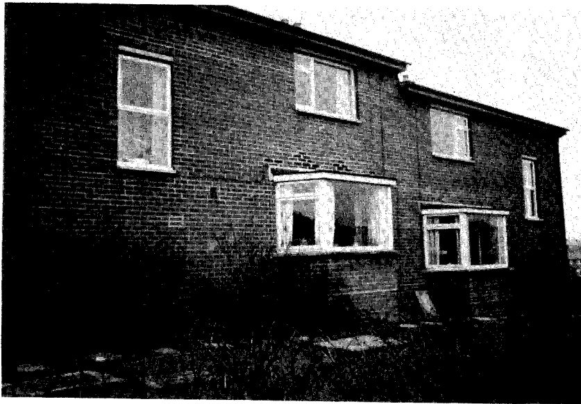
This was the beginning of Peterlee. The house (above) shows evidence of minor subsidence repairs.
