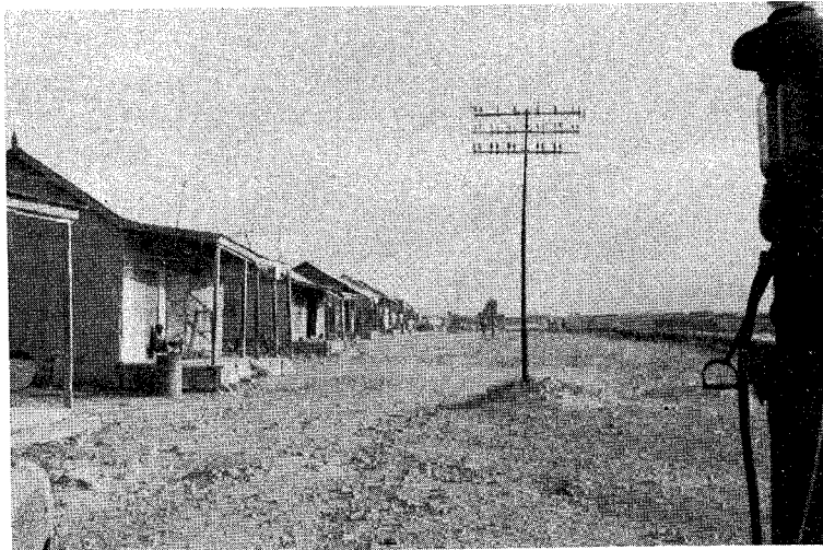
Isiolo, looking south from the gas station
